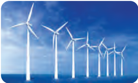
海洋风电塔筒 Offshore wind tower
